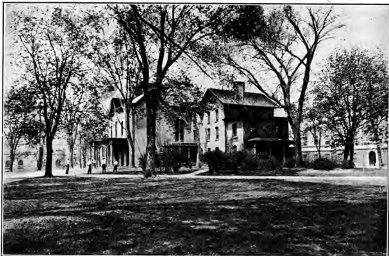
Warren Residence. Dormitory, 1905-1935
