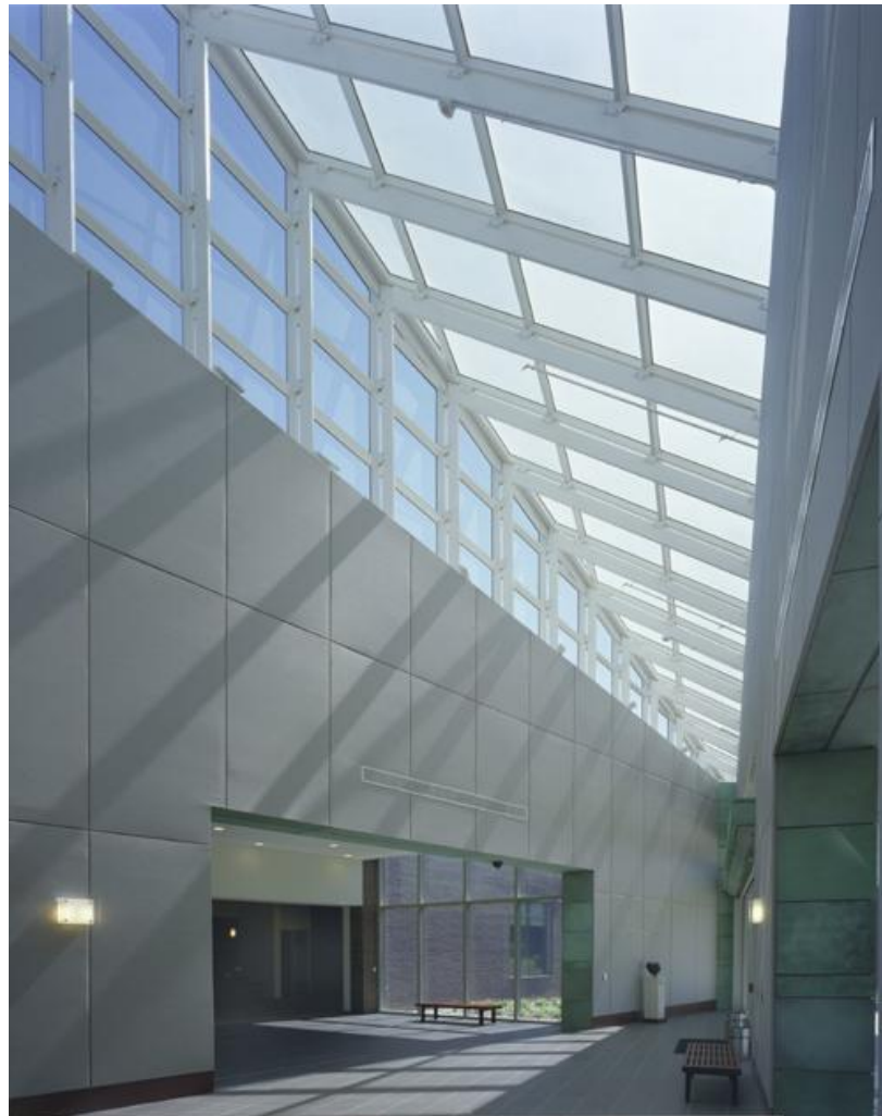
Figure 2: NERL Headquarters. Inside the NERL's Green Building, Research Triangle Park, North Carolina.
